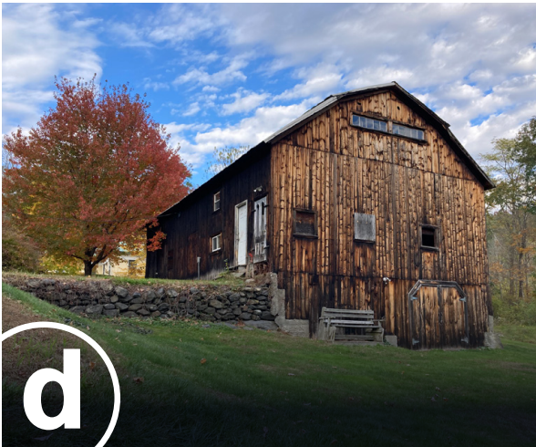
Barn Renovation or Coffeehouse Expansion?
